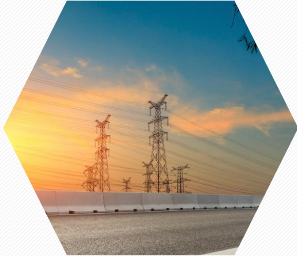
Environment Monitoring System
