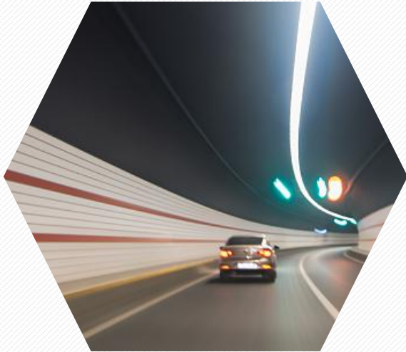
Expressway Tunnel Wireless Patrol System
